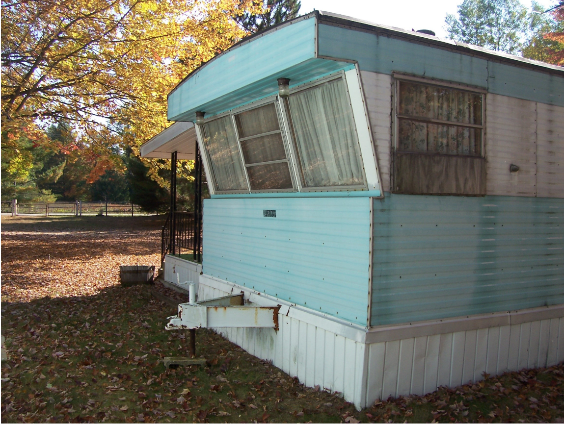
Towing Hitch Still Attached Must Be Removed
