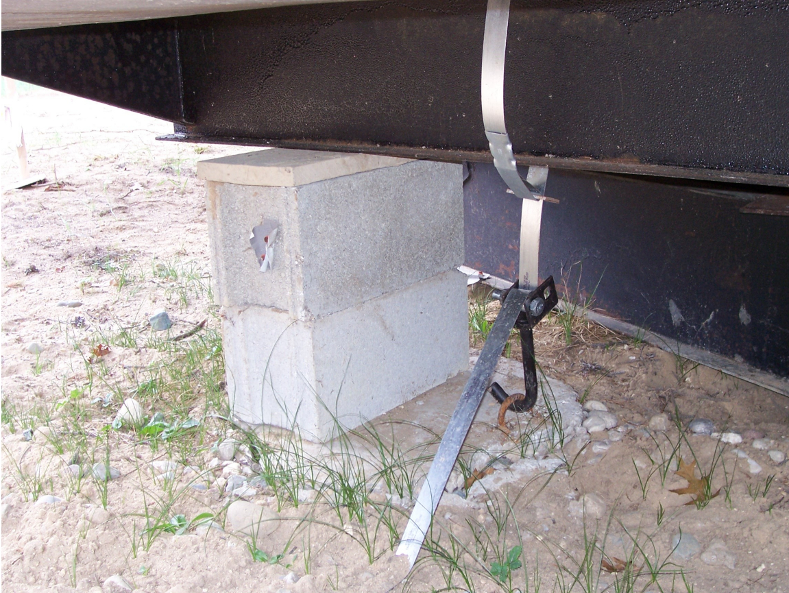
Pier Foundation with Tie-Down
