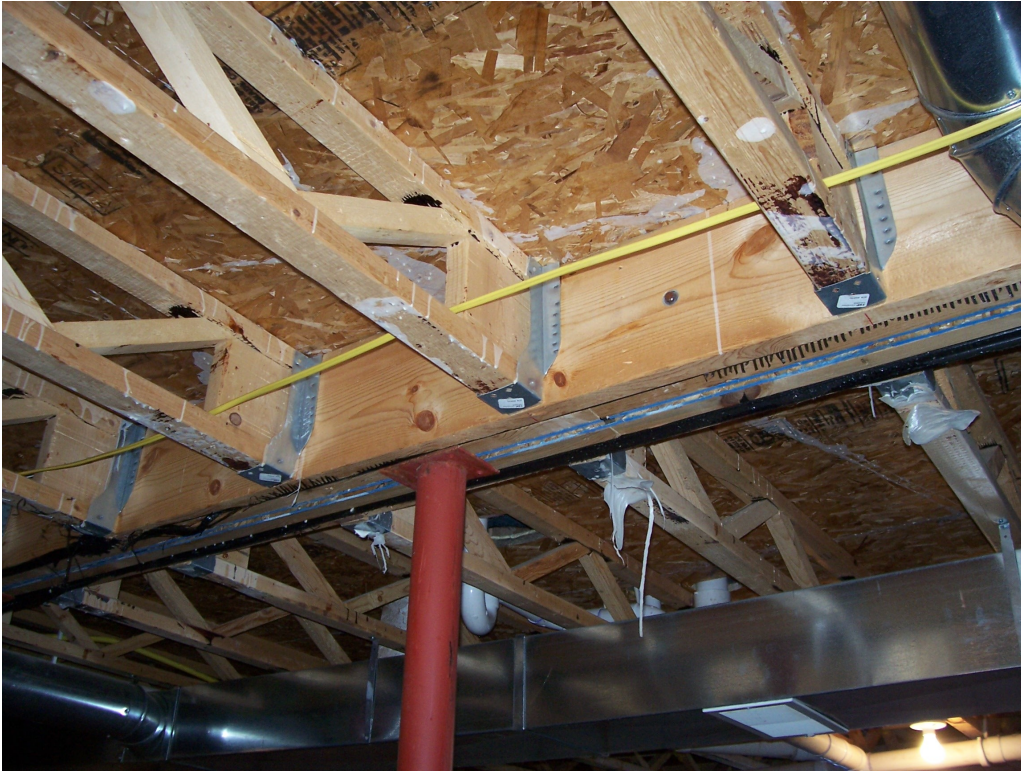
A girder will support floor joist near the center of the house
